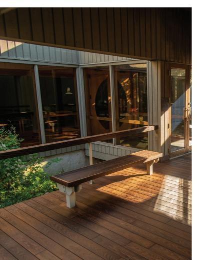
Americana™ Thermally Modified Wood Decking designs are easy to work with. We use standard symmetrical profiles which can be used with off-the-shelf hidden fasteners. You choose which side of the board you see, and with our structural end joint, the deck can be laid like flooring, with joints floating anywhere between joists. Less waste, less time.
