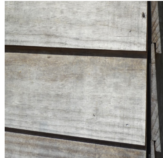
Rough sawn surfaces are more conducive to build-up
