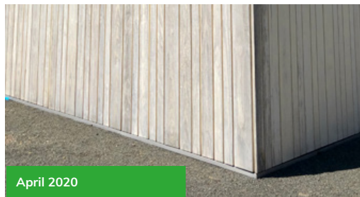
SIDING PROJECT, NORTH AMERICA
