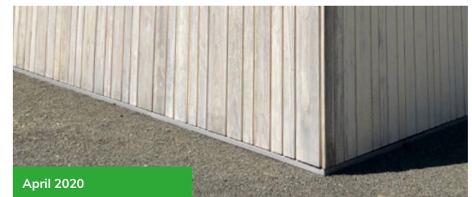
SIDING PROJECT, NORTH AMERICA
