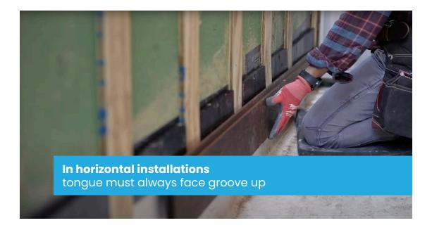
Use furring strips 1" x 2" (per local codes), maximum 16" apart, on top of sheathing\* and house wrap. In horizontal installations, tongue must always face up.
