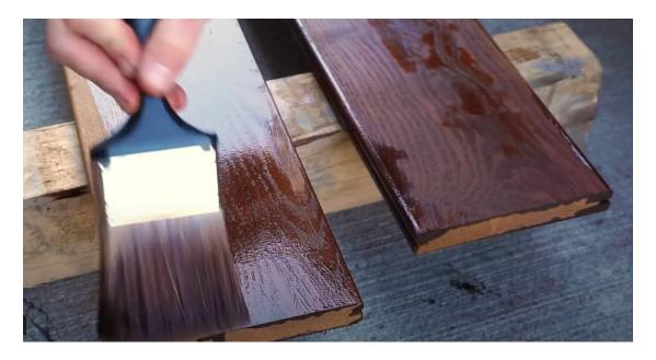
Finishes - For best results, apply Cutek Clear to all sides before installation (or opt for factory-applied Cutek). To maintain or alter the color, apply another coat of Cutek + colortone of your choice on visible surfaces after installation.
